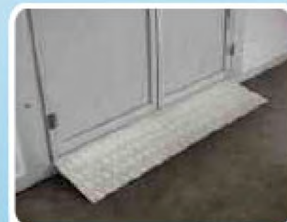
门口斜板 entrance ramp
