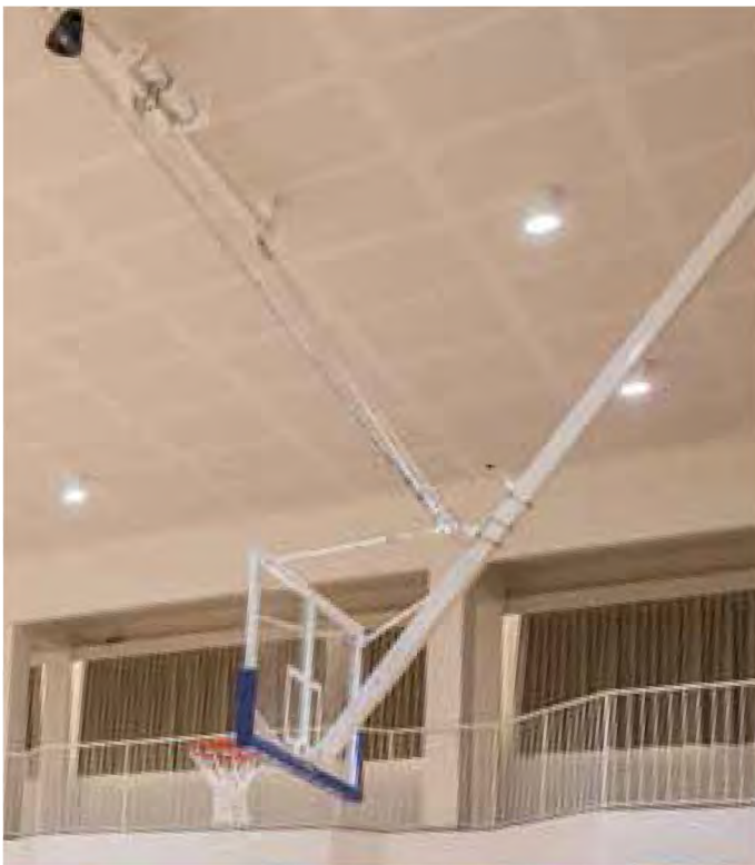
750 - Ceiling suspended goal with fixed height frame.
