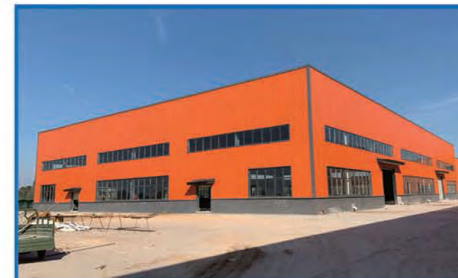
WAREHOUSE/WORKSHOP 仓库/厂房
