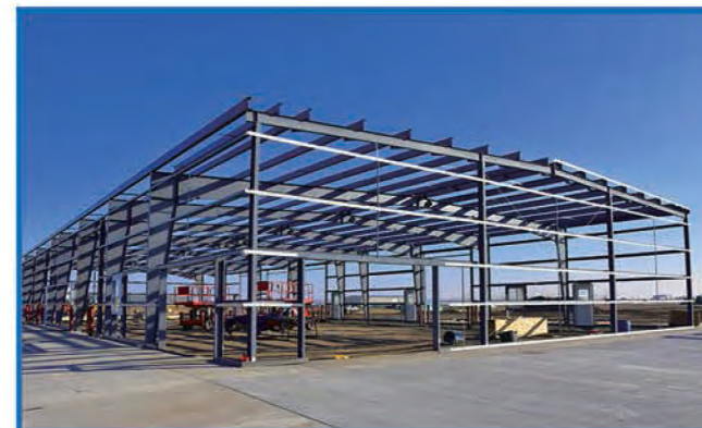
STEEL STRUCTURE 钢结构
