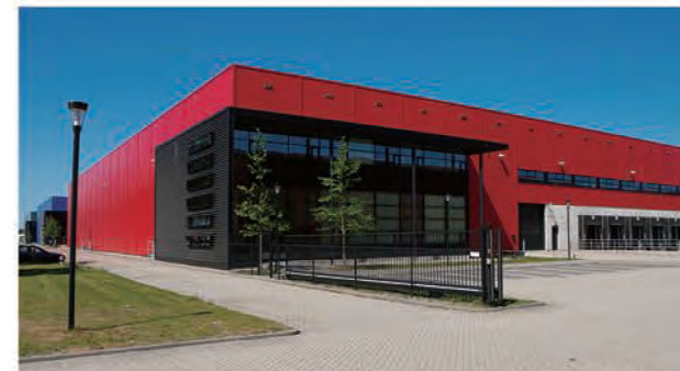
Warehouse/Workshop 仓库/厂房
