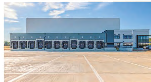
Clean/Cold Room 净化室/冷库
