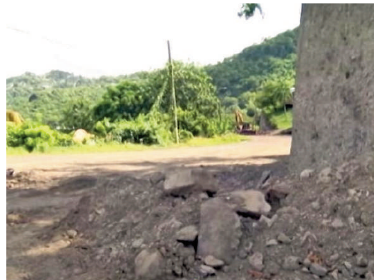
Construction work is still ongoing in the roadway known as Woburn/Cliff
