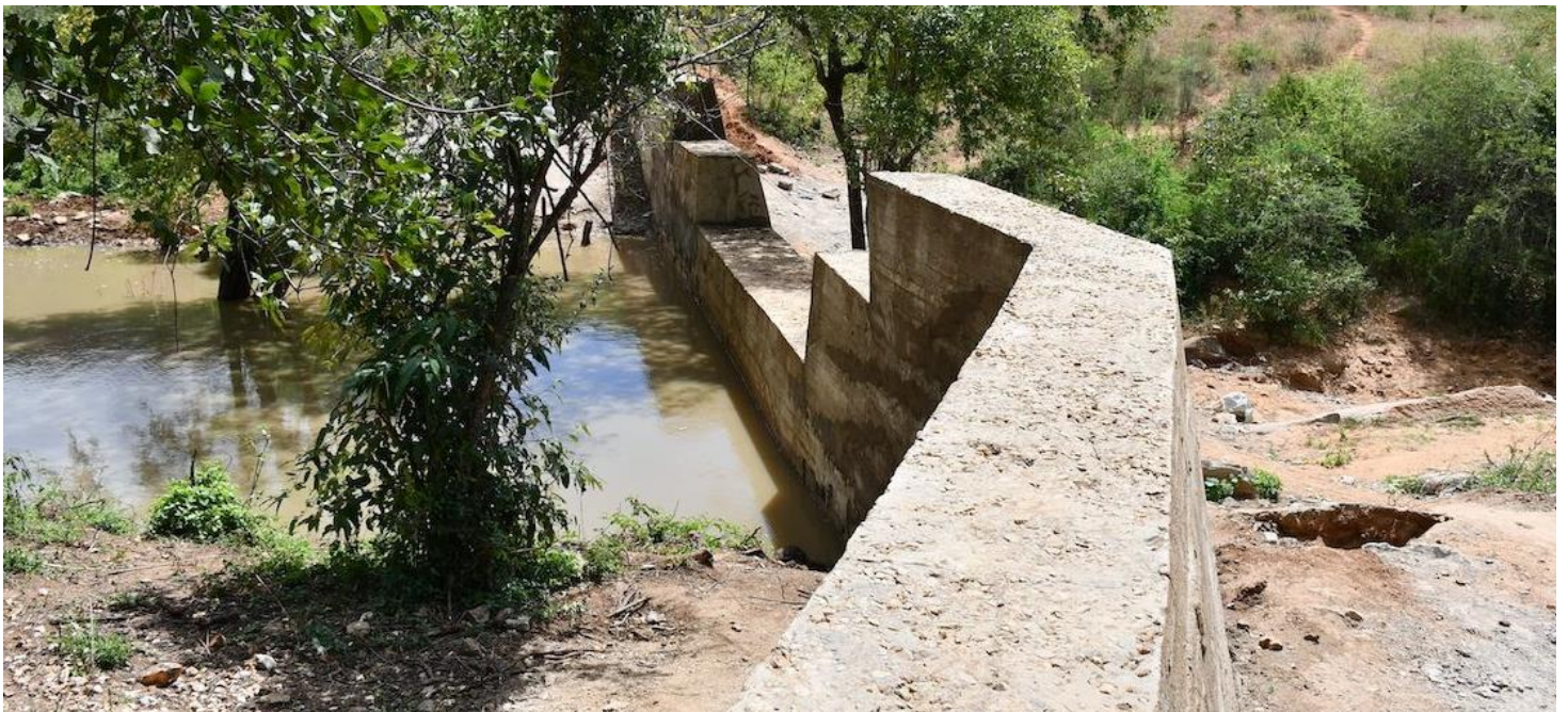
The finished sand dam
