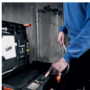
Automatic tightness test
