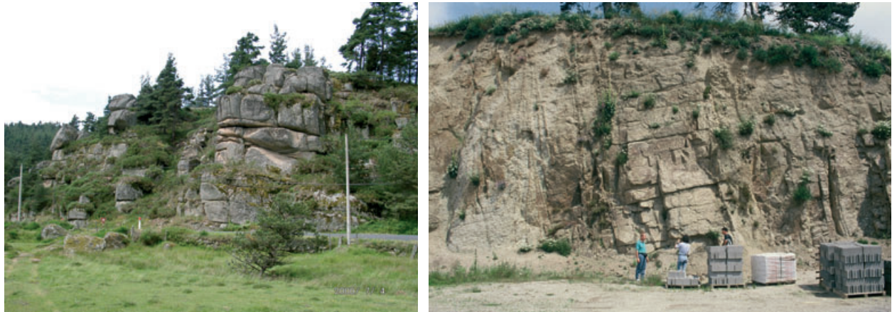
Fig. 2 The fissured horizon in granites (Lozère, France) outcropping (left: near the village of Serverette; the ~5 m high phone pole gives the scale) and in a former quarry (right: near the village of Rieutort de Randon).
