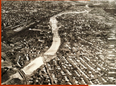
Aerial view of I-95 under construction in the Spring of 1956.
