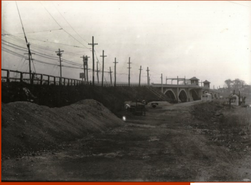
Washington Bridge under construction in 1921.
