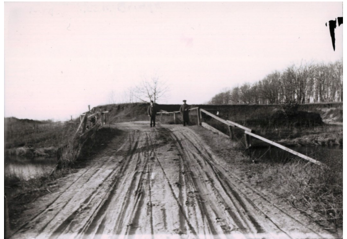
Neck Creek Bridge c 1895
