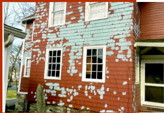
Judson House being prepared for painting. Photo courtesy of Jim Shannon.
