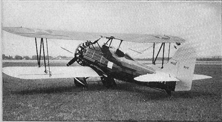
The SU-2, produced in 1933, was a two-place scout plane with a speed of 170 m.p.h.
