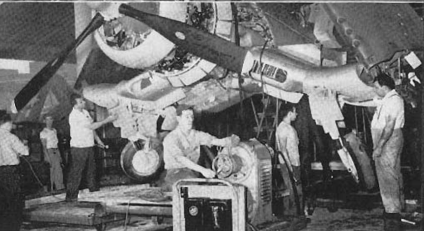
Landing gear is retracted as workers carefully check Corsair's hydraulic system.
