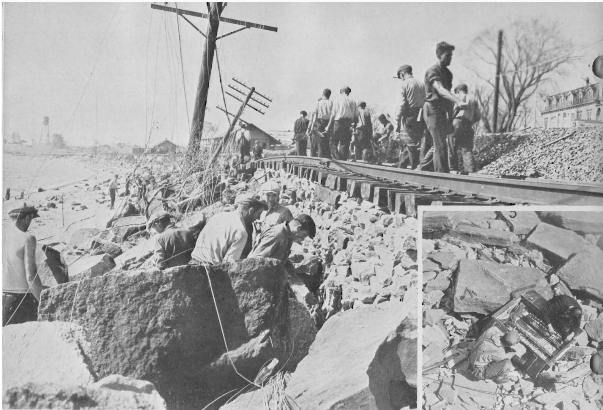
RECONSTRUCTION begins . . . communications must first be established . . . wires untangled . . .
