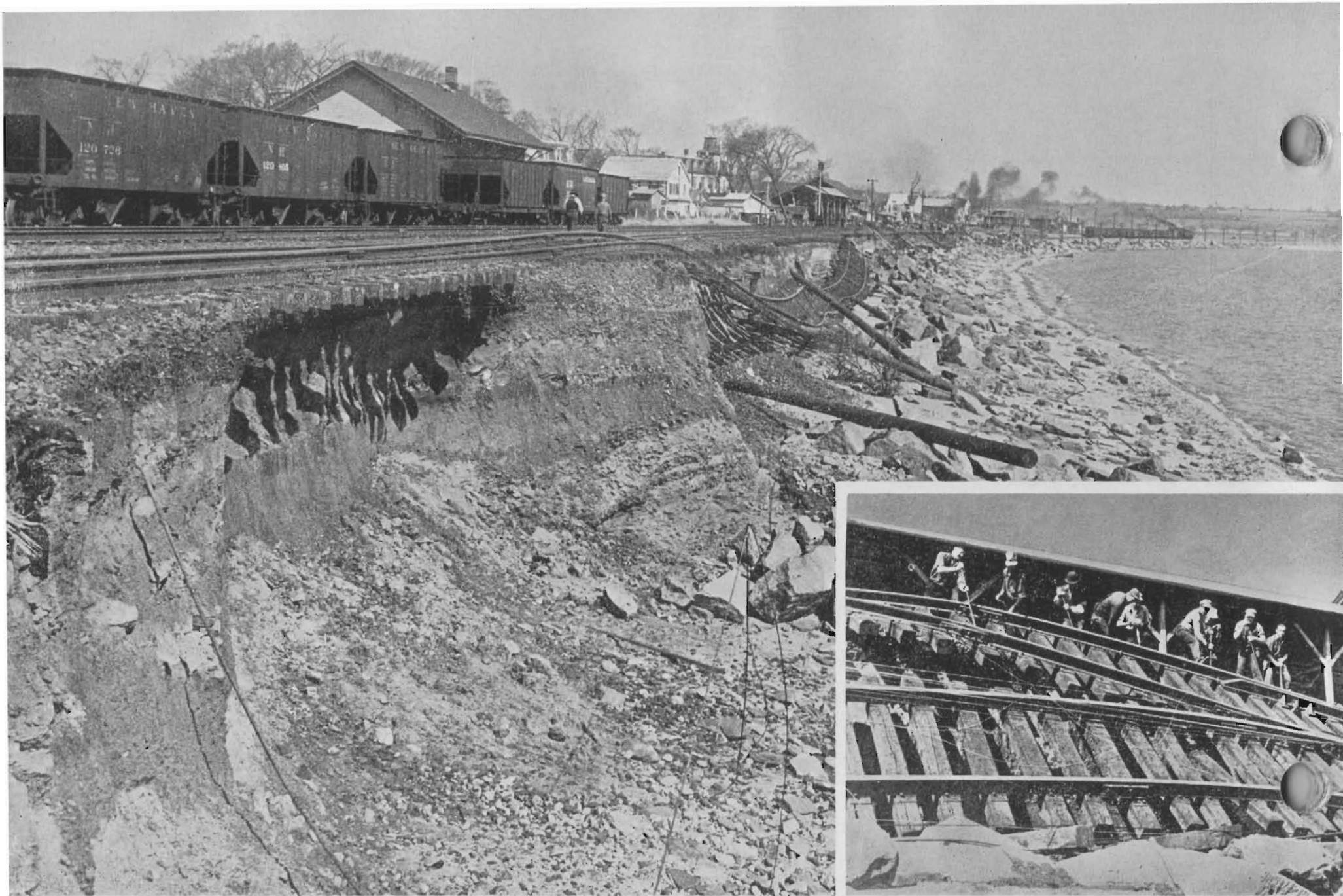
MAN-POWER ALONE can right these twisted rails . . . foot by foot they must be jacked up and underpinned
