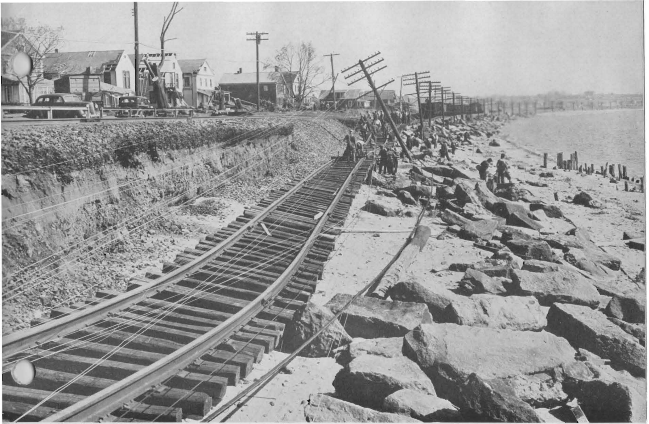
with rip-rap . . . followed by tons of fill . . . a procedure more difficult than laying new track.
