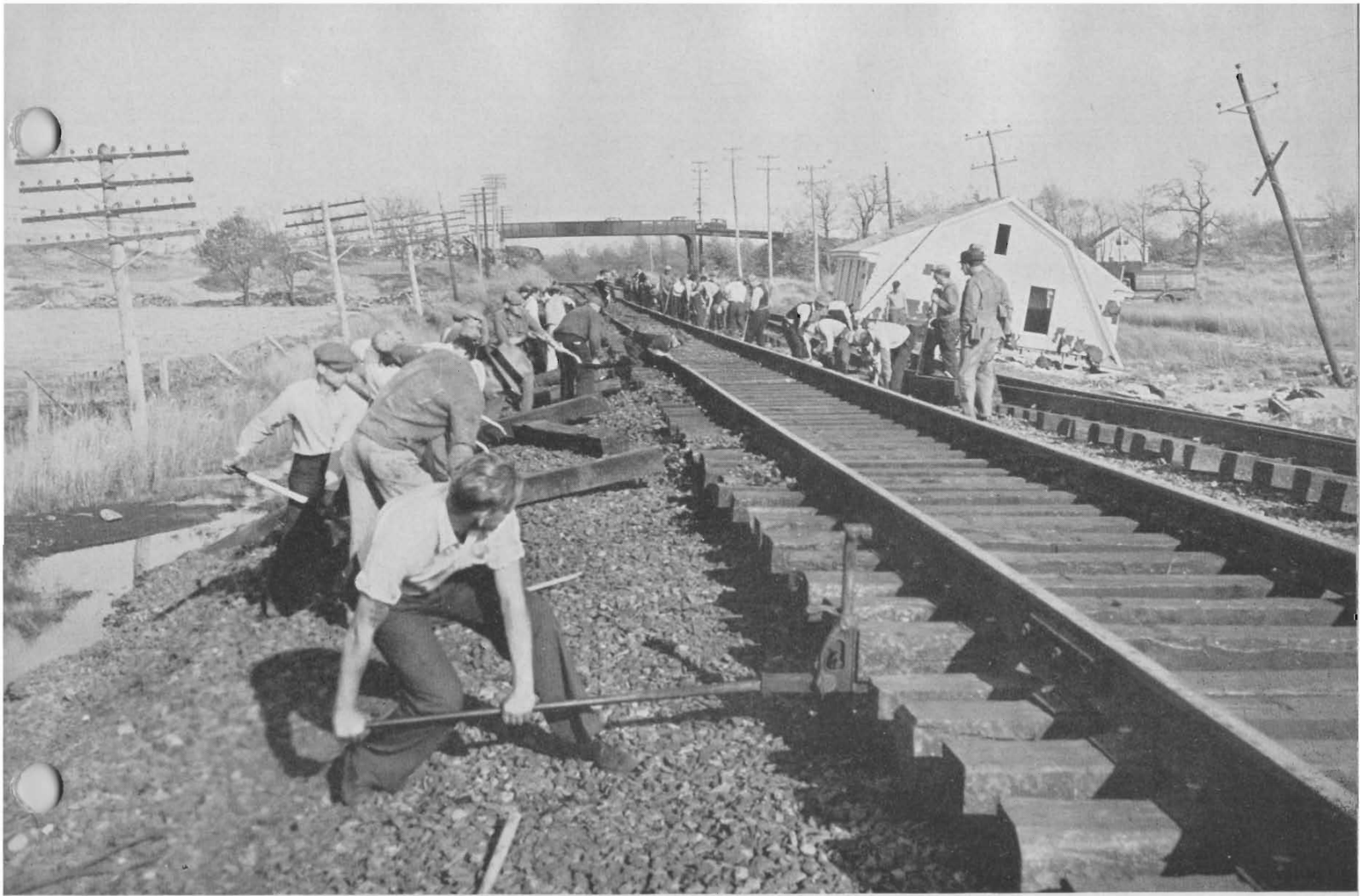
former level and filled in with crushed stone.
