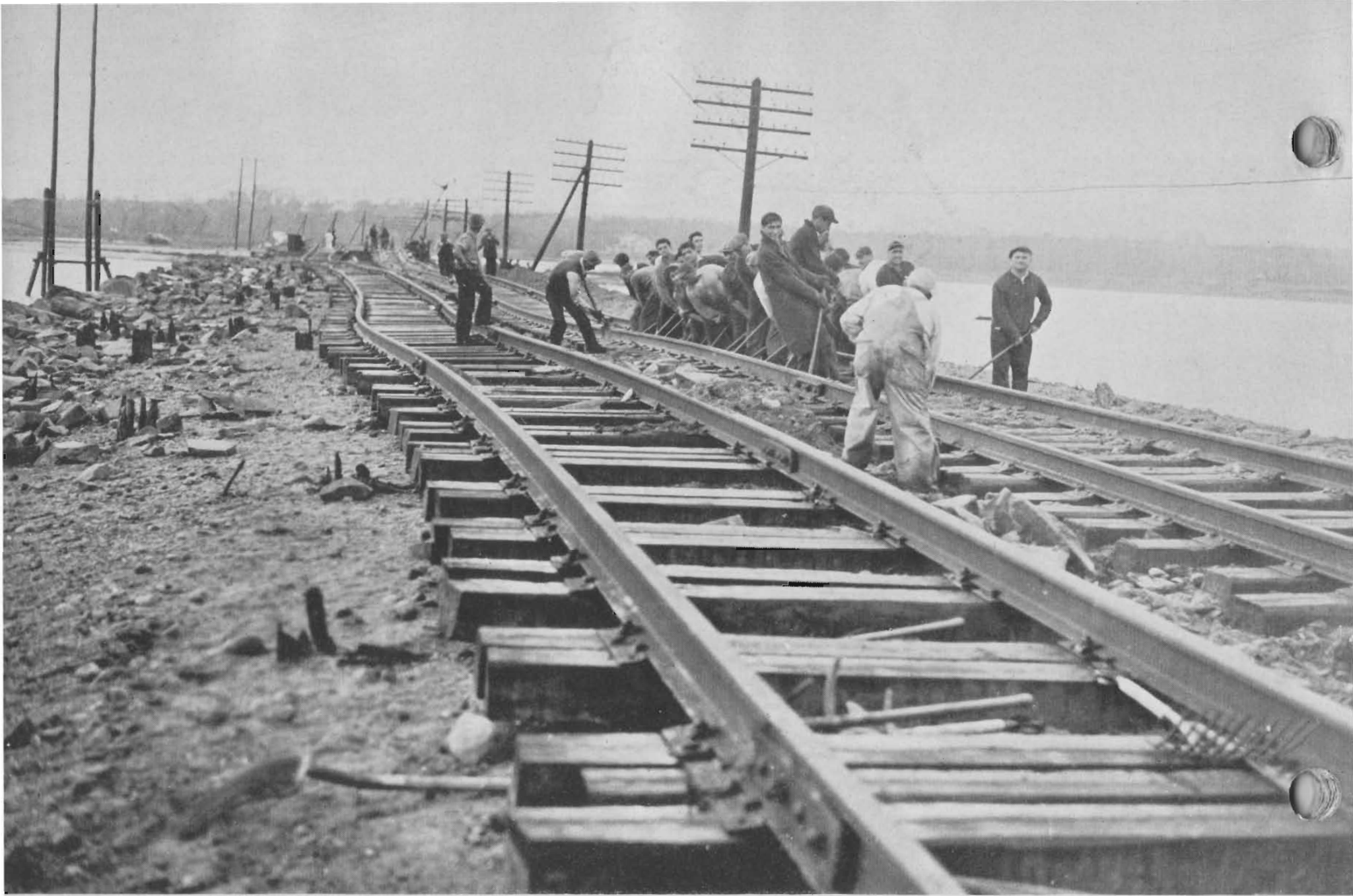
Taking out the kinks in the tracks is a matter of mass cooperation . . . after which the tracks are jacked up to their
