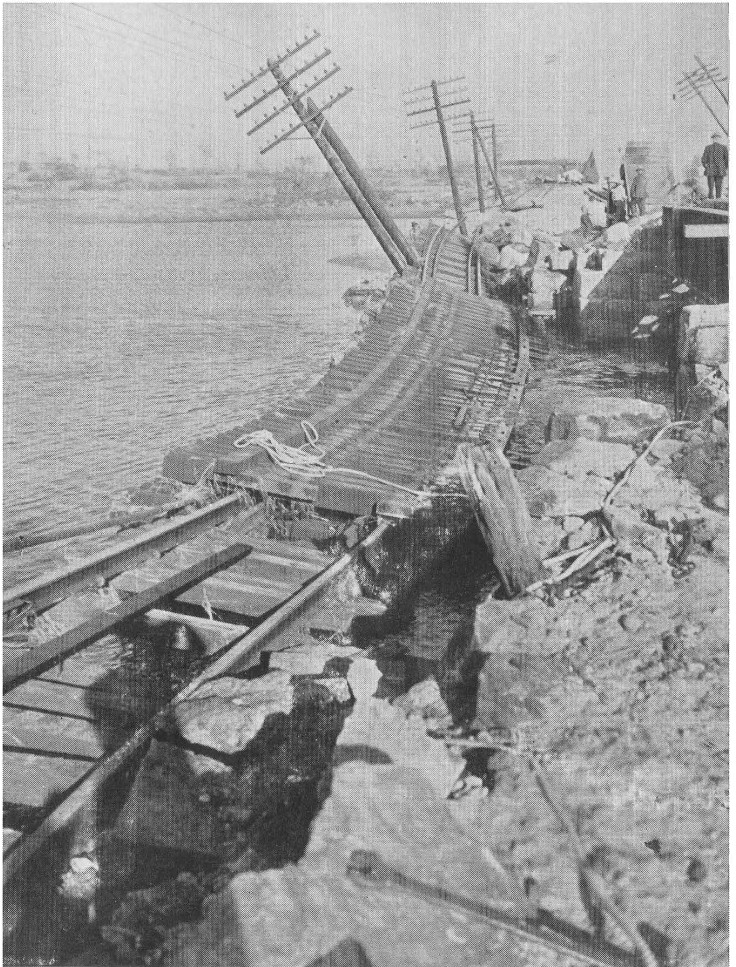
. . . tracks and platform lifted completely off bridge.
