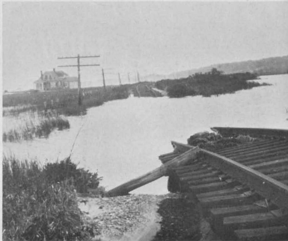
WOODS HOLE branch from Bourne to Falmouth was under sand and water with bridges and culverts out.
