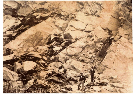
Boothe Brothers at the rock quarry in the present day Roosevelt Forest c 1900
