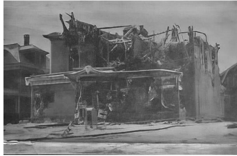
All that is left of the Stratford post office, built shortly after the Civil War at a total cost of $25,000.
