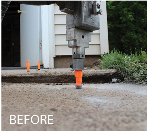
Prepping holes for mud jacking
