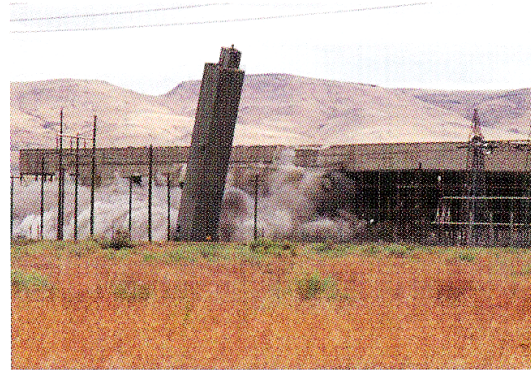
Demolition of surplus contaminated facilities
