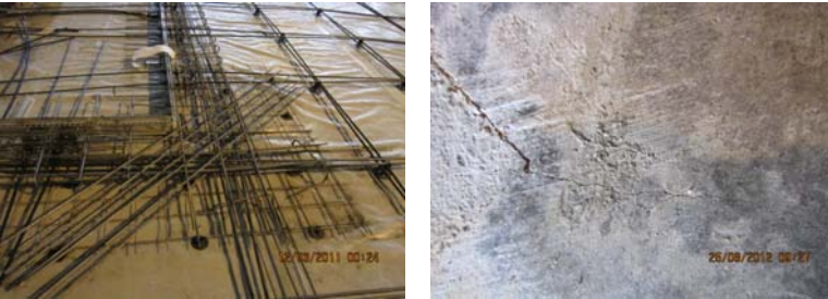
Trim bars at joint
