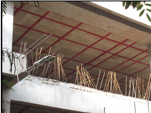
Marking of tendons at slab soffit
