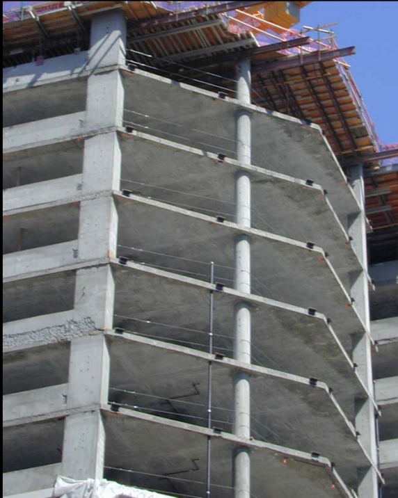
Close up of a flat slab post-tensioned concrete frame in San Francisco
