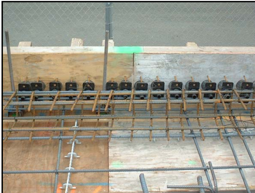
Arrangement of anti- bursting reinforcement at live ends of grouped tendons, prior to installation of tendons
