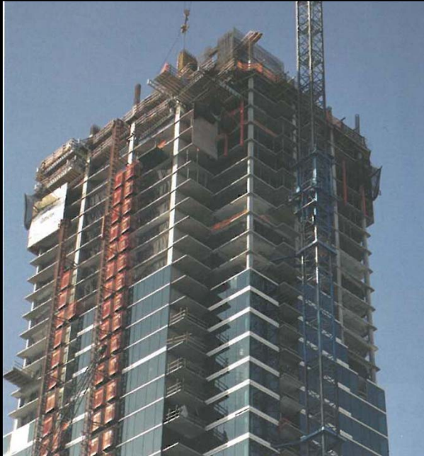
Rincon Tower San Francisco, California Post-tensioned flat slab construction
