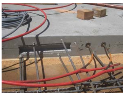
With intermediate stressing; finished on one side
