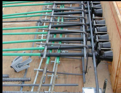
Stressing End Detail for Grouped Tendons
