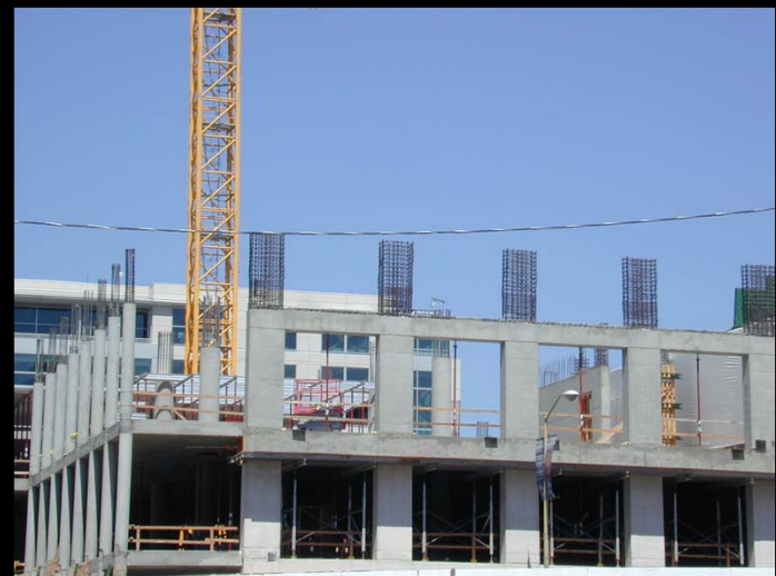
Concrete frame under construction in San Francisco
