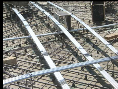
Examples of closely bundled and adequately spaced grouted tendons
