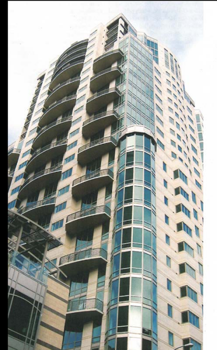
The Metropolitan; San Francisco Post-tensioned flat slab construction
