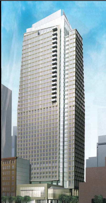
St Regis; San Francisco Post-tensioned flat slab construction
