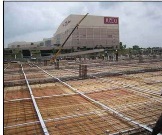
Construction with widely spaced tendons (Egypt)
