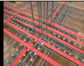
Slab construction with unbonded tendons. Neither ACI, nor EC2 require strength check at initiation of cracking (P998)
