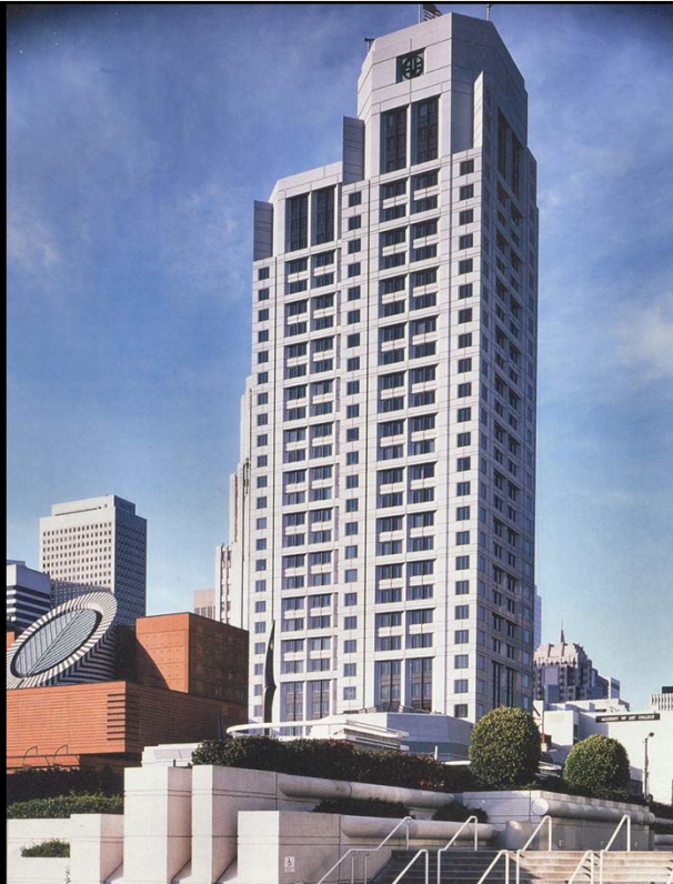
W Hotel, San Francisco, California post-tensioned flat slab floors
