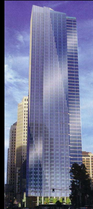
301 Mission Street San Francisco, California post-tensioned flat slab construction
