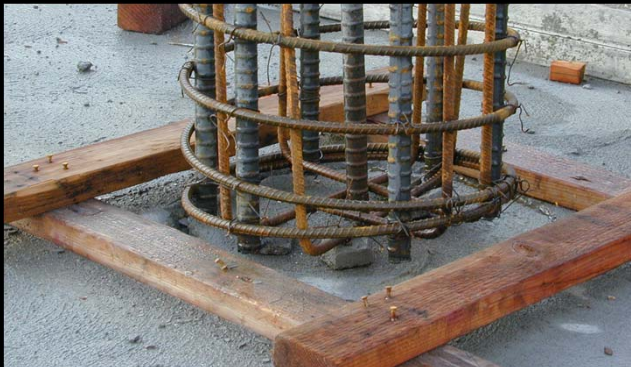
Upper column reinforcement is placed on top of slab
