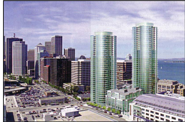
Infinity Towers (36 story + 4 underground) San Francisco, California
