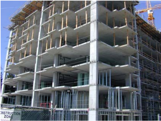
Upper levels of multi-story buildings do not generally require crack mitigation measures
