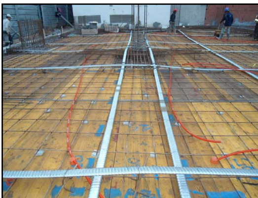
Sparsely positioned tendons (bonded system; Morocco)
