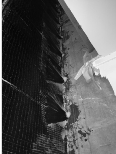
Additional example of column confinement utilising composite anchors
