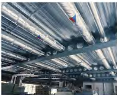
Sizes of composite cellular beams as secondary beams (IPE/HE sections in S355 steel)
