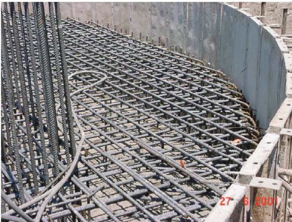
Footing reinforcement and mould
