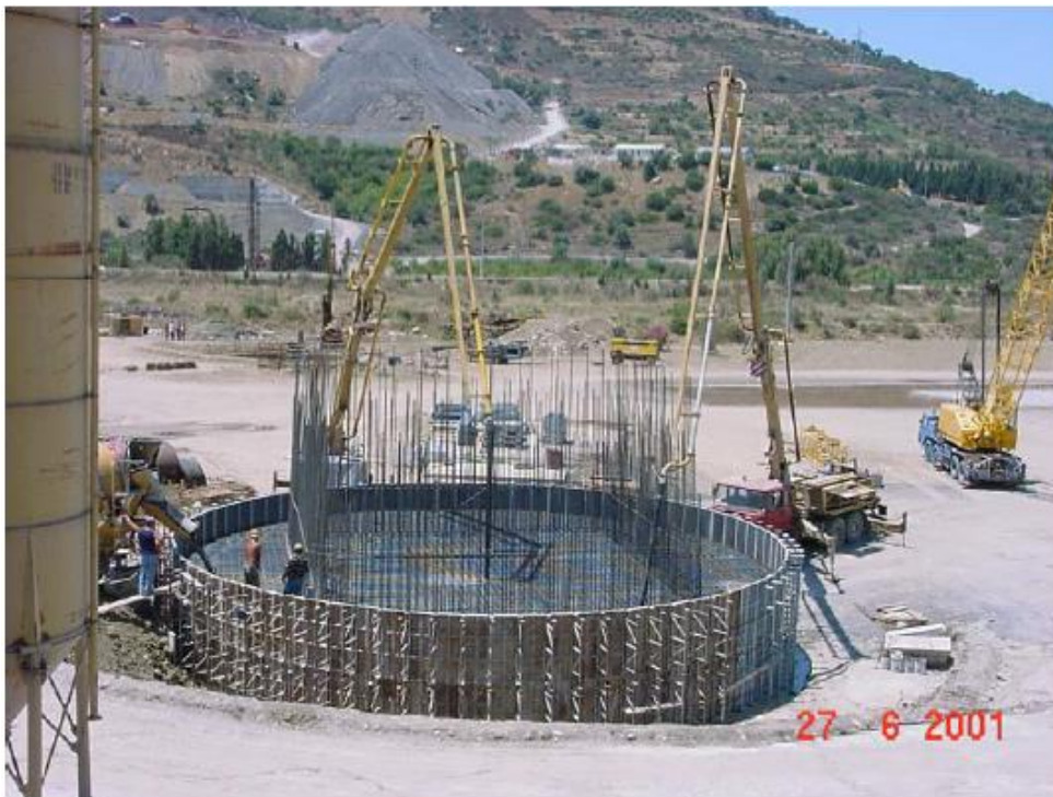
Concreting of the footing
