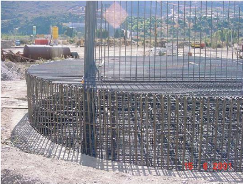
Footing reinforcement 2
