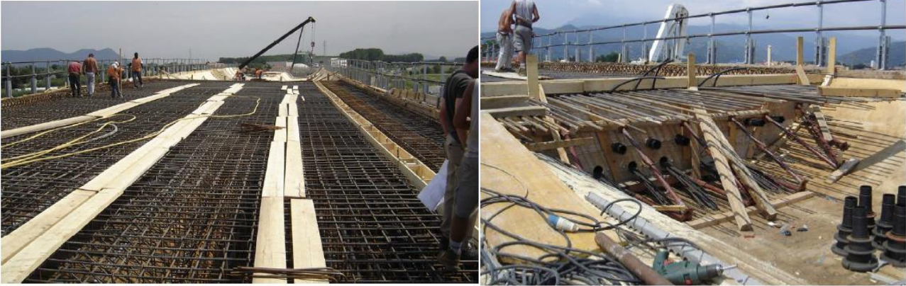
Reinforcement just before concreting
