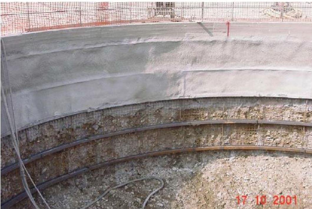
Hopping before spritzbeton
