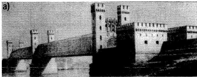
a) Marienburg Bridge on Nogat River (Germany, 1857)
