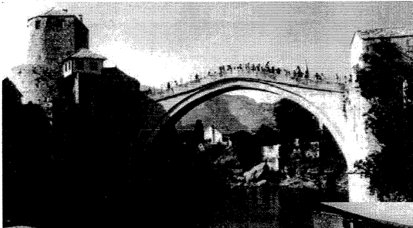
Roman Bridge in Mostar span: 29m depth: 25m ( Jugoslavia, ~ 1500 on old roman ruins, rebuilt in 2004)
