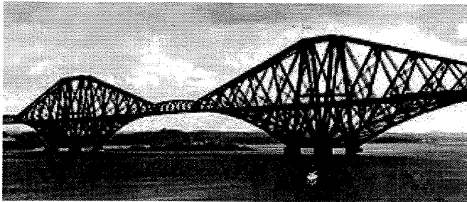
Firth of Forth bridge (1889 ÷ 1890) max span: 521m
