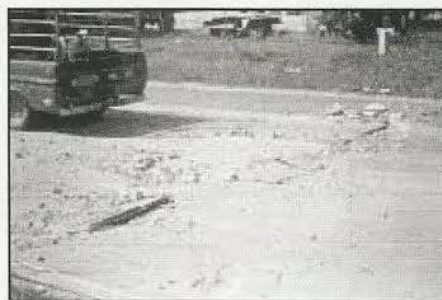
FIGURE 76 Distress Type JCP 11—A Blowup
