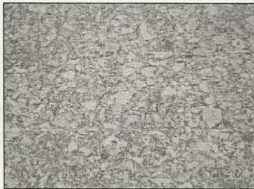
FIGURE 39 Distress Type ACP 12—Polished Aggregate
