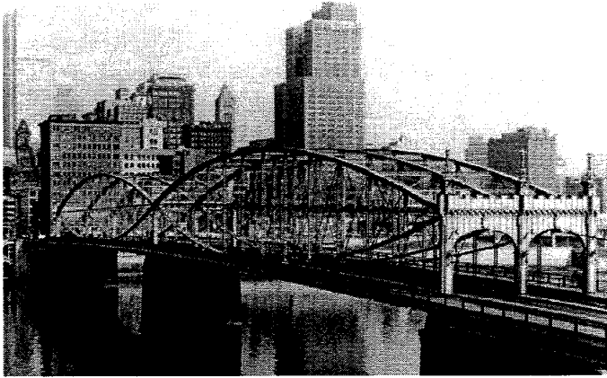
Smithfield Street bridge max span: 109m (Pittsburgh, 1883)
