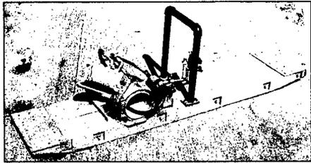
Figure 4. A small skid with a compressed air vibrator to accomplish vibratory locomotion.
