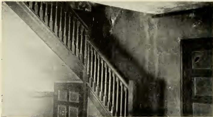
Stairway in Huggins House
