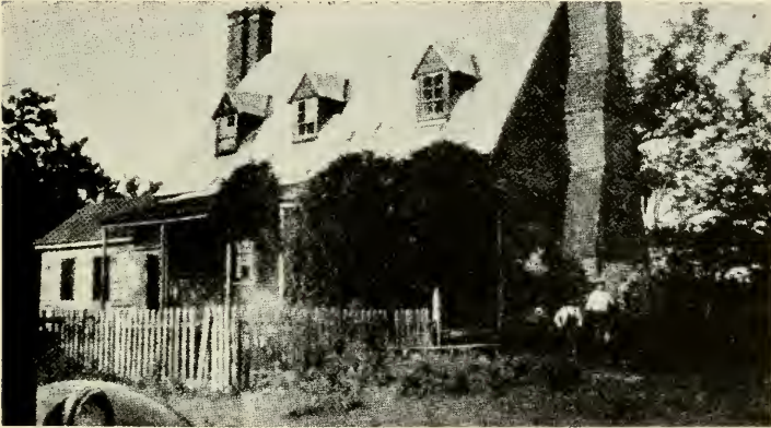
Wishart House before roof was changed
