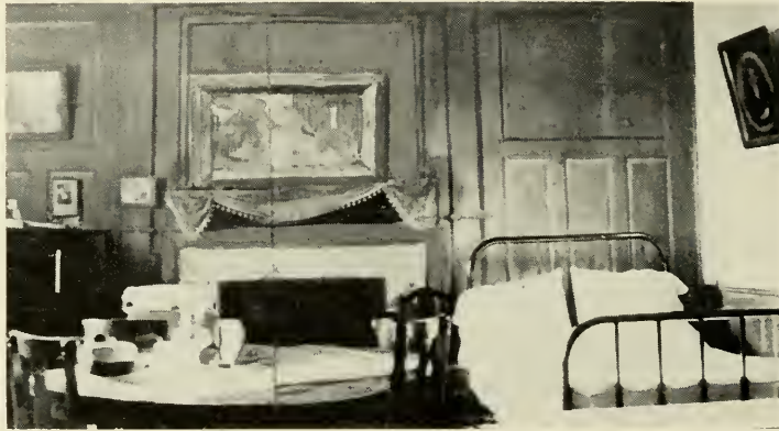
Interior of south room in Shipp Home
