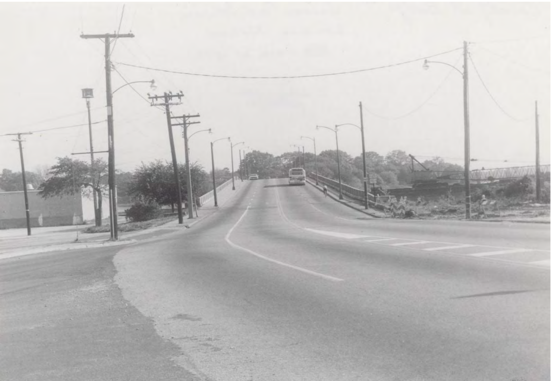
Granby Street Bridge looking North - 1977
