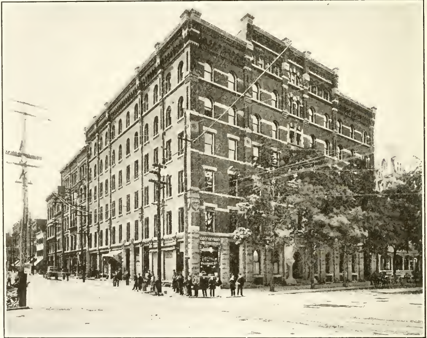
HOLLENBACK COAL EXCHANGE—1890
