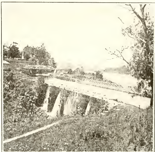
MILL CREEK AQUEDUCT.
