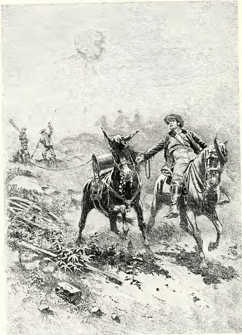
STRINGING TELEGRAPH WIRES UNDER FIRE
