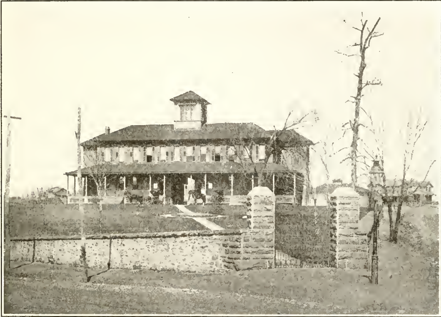
ORIGINAL BUILDING OF CITY HOSPITAL
