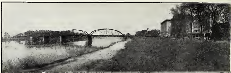
View North-east from near the Site of Fort Wyoming in 1902.
