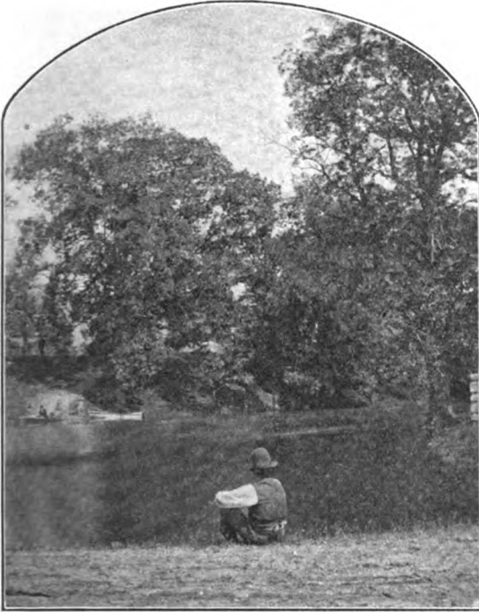
ABRAHAM'S CREEK, Near the "stone-arched bridge," in 1878.
