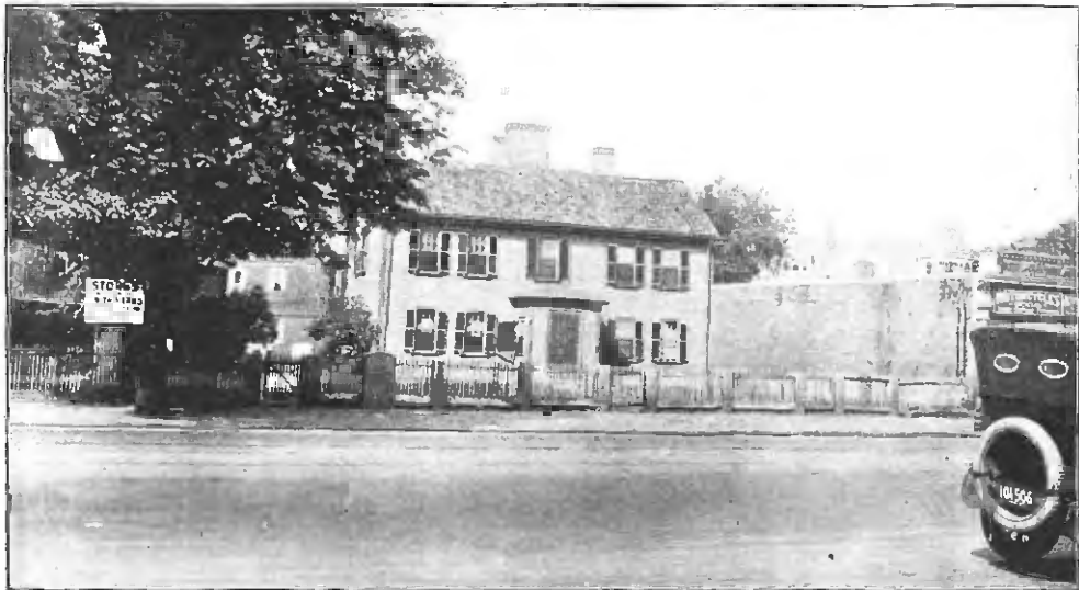
The Watson House, Massachusetts Avenue, Cambridge. Demolished in 1921.
