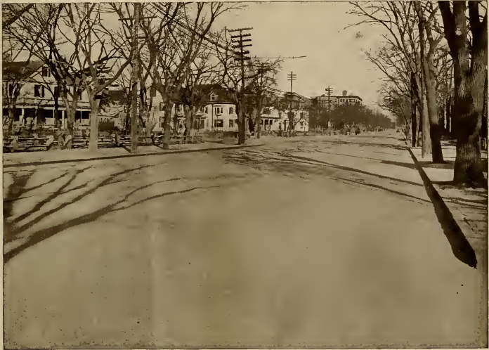
MASSACHUSETTS AVENUE LOOKING NORTH FROM WATERHOUSE STREET Courtesy of Warren Bros. Co.
