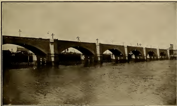
THE VIADUCT (Over the Charles; from Boston to East Cambridge)
