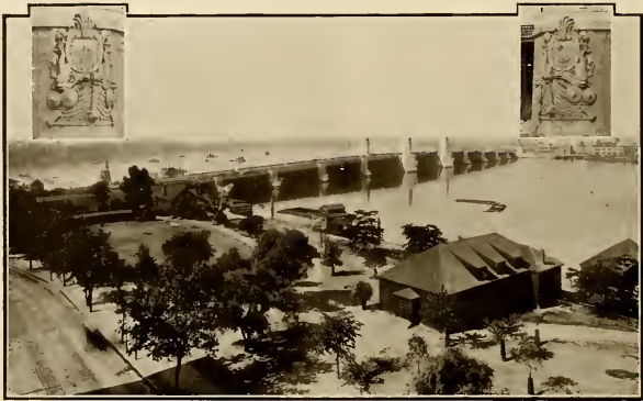
THE NEW CAMBRIDGE BRIDGE
