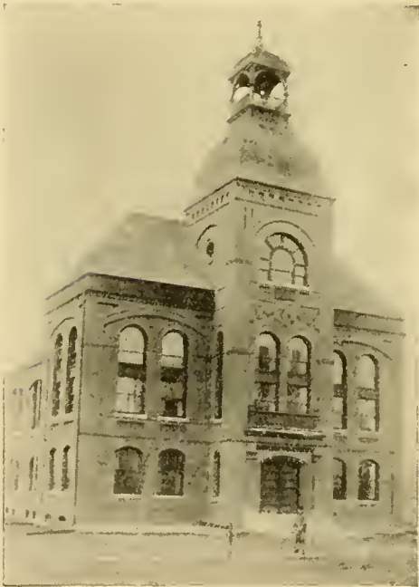
Court House, Lancaster
