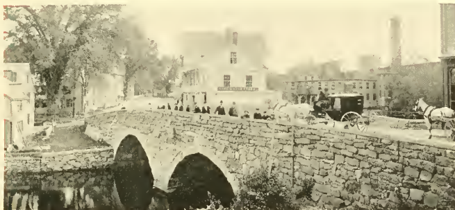
THE CHOATE BRIDGE, 1837. (Lower Side.)
