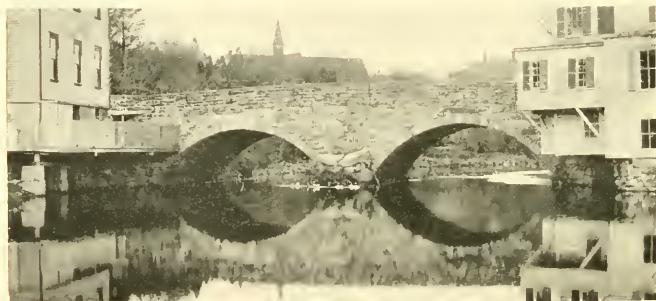
THE CHOATE BRIDGE, 1764 (Upper side)
